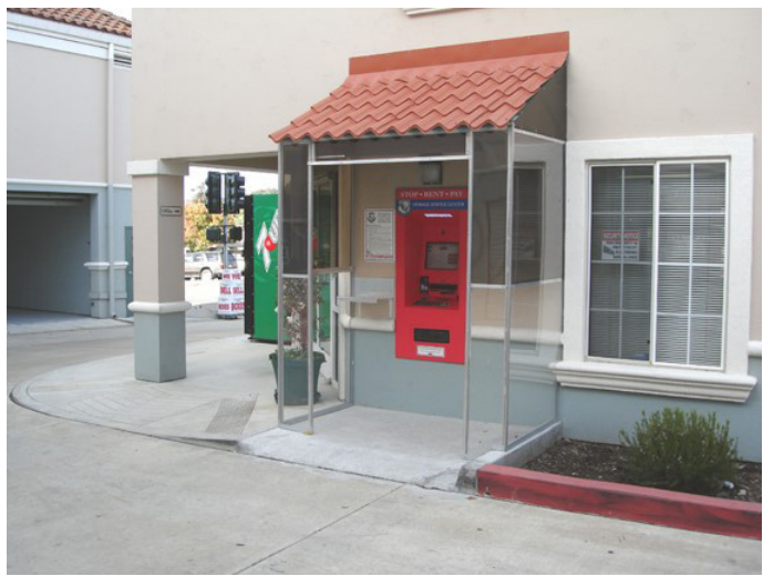
Figure 8: Vestibule Enclosure Installation for a through-the-wall style installation
